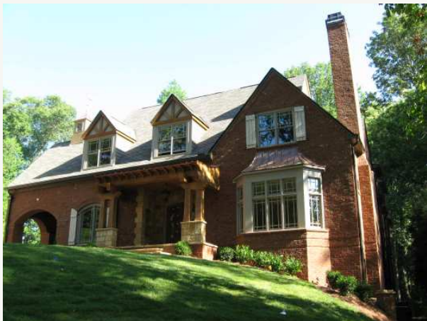
4594 East Conway Drive, New home by Canonbury Homes $1,895,000 - Beautiful old world style
